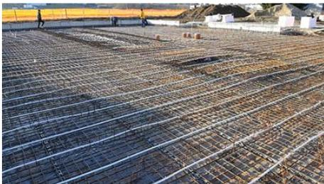
Electric heating wires will activate the concrete foundation of the building in the future.
